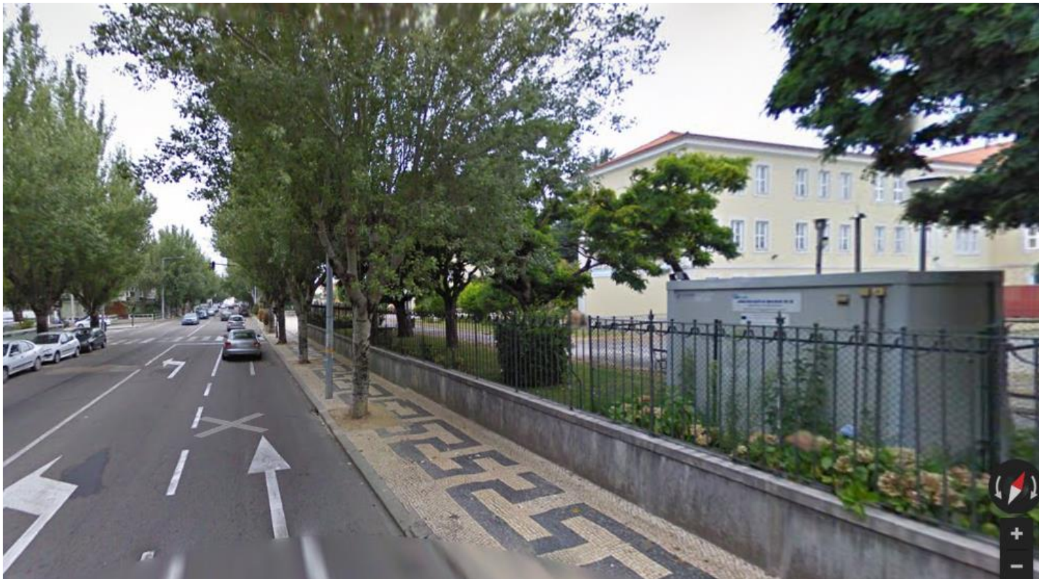
(Aveiro/Av.25Abril - Air Quality monitoring station)
