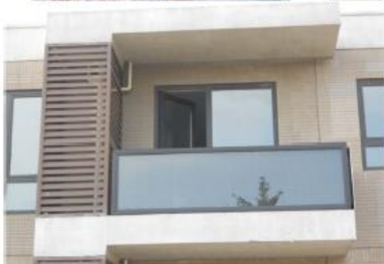
Solar collectors act as balcony railings of the building, Beijing, China
