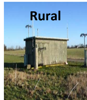
AQ monitoring station by Aarhus University, DK
