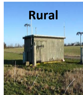
AQ monitoring station by Aarhus University, DK
