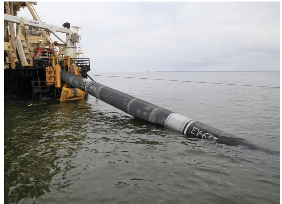
Monitoring of leakage from underwater pipelines
